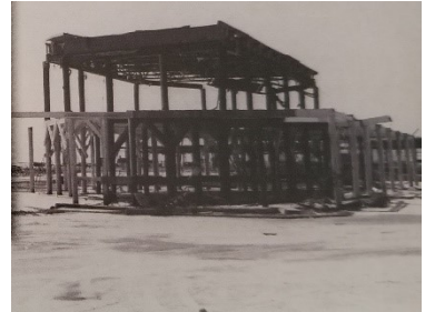
Gulfport Yacht Club 1969 after Hurricane Camile
